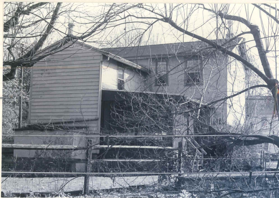
NW-rear, wood shed, porch (GHL: 91-11/3)
