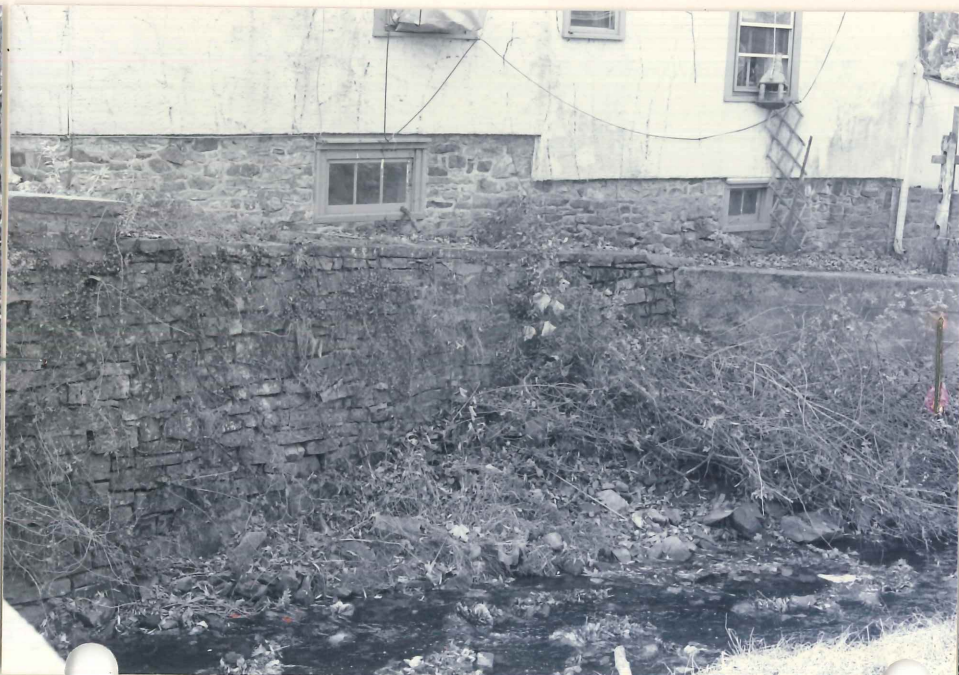
NE-exterior detail of stone wall (GHL:91-11/13)
