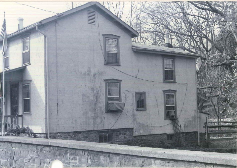
NE-gable end from bridge (GHL: 91-11/12)
