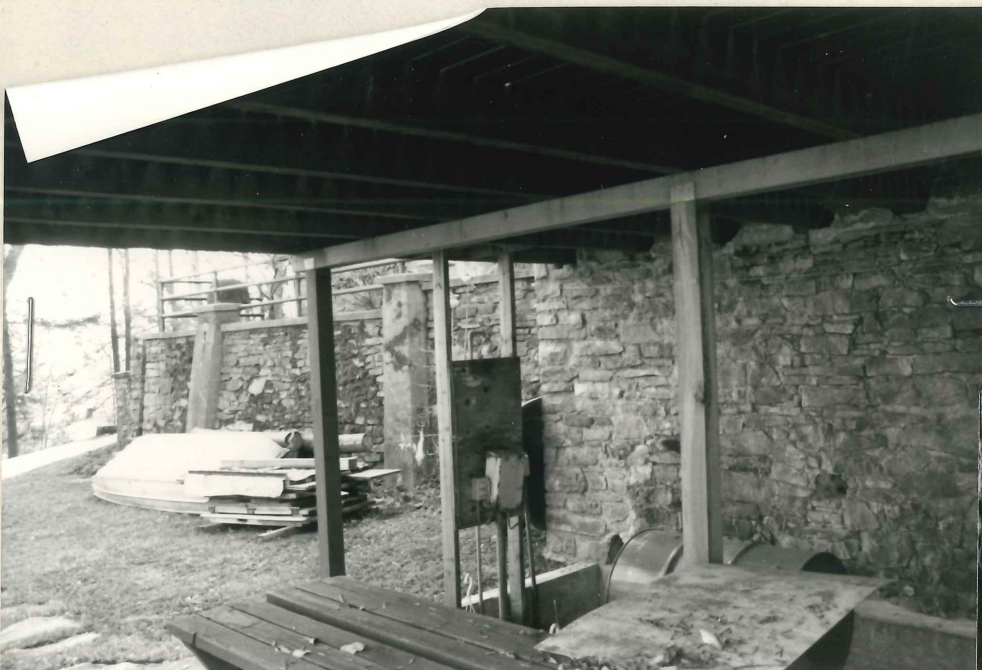
Carriage Hse. walls under deck, air pressure tank (11/14/91) (KAA: 91-14/ 11A-12)
