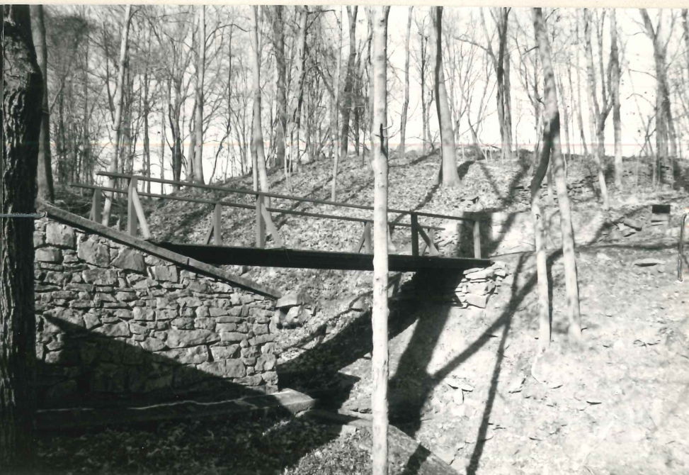
// Rear yard, stone retaining wall & bridge (11/14/91) (KAA: 91-14/ 12A-13)
